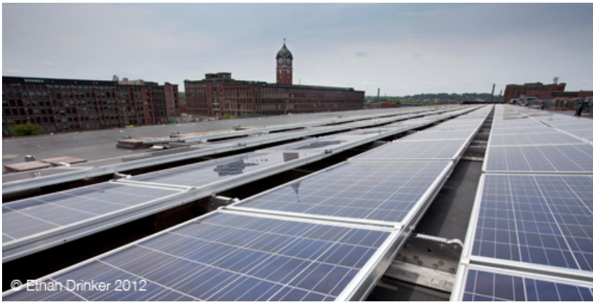
Figure 14: Union Crossing Building 9 Lawrence, MA Coldham and Hartman
