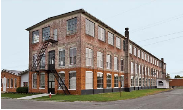
Figure 19: The Cracker Factory Miles and May Furniture Works Geneva, NY Amy and Brandon Phillips
