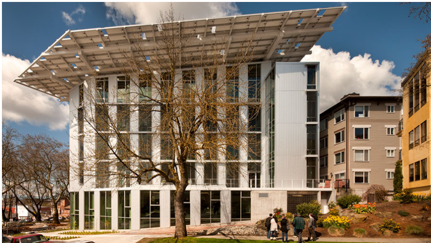
Figure 4: Bullitt Center Seattle, WA Miller Hull
