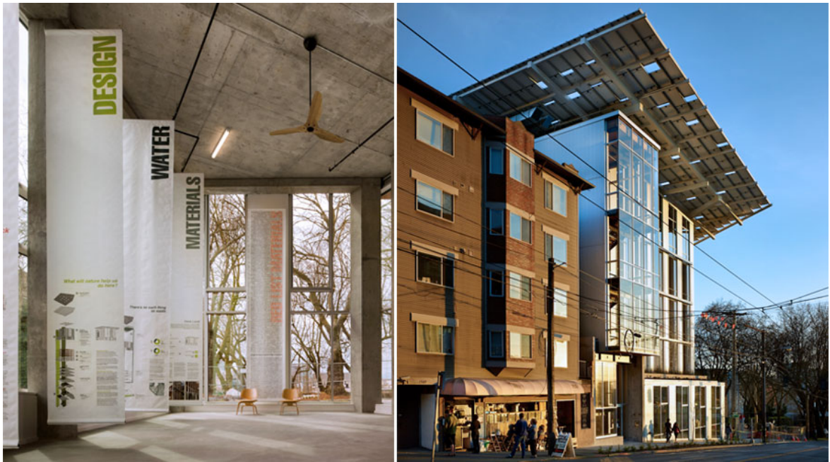
Figure 5: Bullitt Center Seattle, WA Miller Hull
